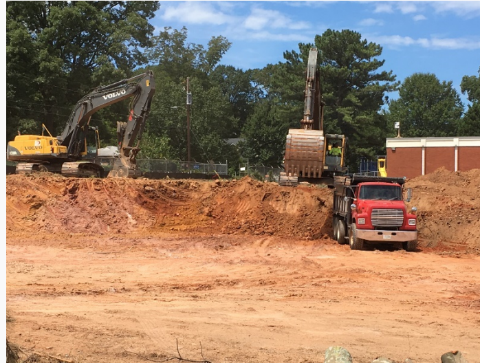
Cut for installation of retaining wall footing
