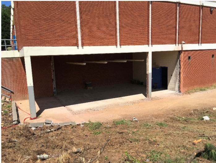
Demolition of lower level for retaining wall
