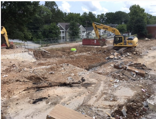
Slab on Grade Removal
